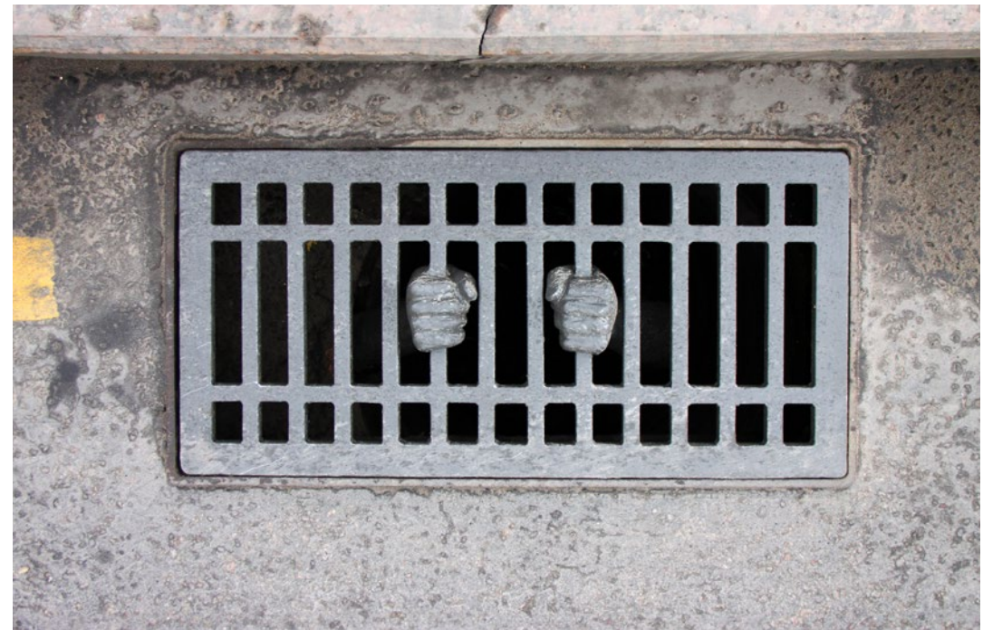
View from the sidewalk
